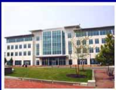
Ferry Terminal Office Building (2007)
