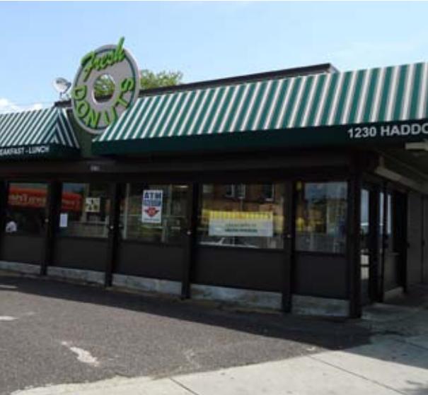
PBCIP used NRTC funds to renovate local business facades to help attract more people and businesses to Camden’s long- disinvested Haddon Ave corridor.
