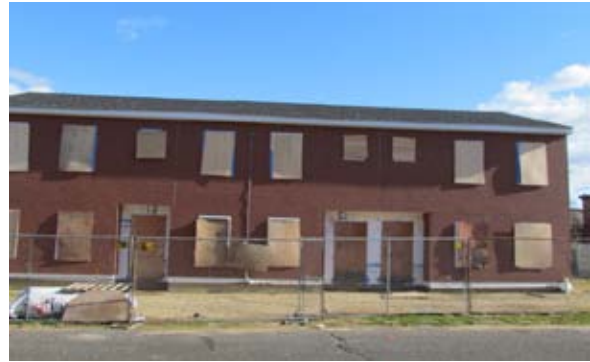
Top: Six new residential apartments under construction in Camden’s Cooper University neighborhood thanks to Habitat for Humanity and NRTC investment.
